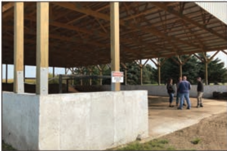
Left, from left: Shirley and Kevin Klaphake told Mike Hemmann, a Stearns County-based NRCS civil engineering technician, and Stearns County SWCD Project Management Supervisor Nathan Hylla how a newly constructed, roofed stacking slab built to store 12 months of poultry litter fit into their operation. Right: Meyer, seen here shortly after a 40-by-100-foot covered stacking slab was constructed near the poultry barn on his Lake Henry Township farm, said having 12 months' storage made it possible to incorporate that nitrogen source in the fall.
